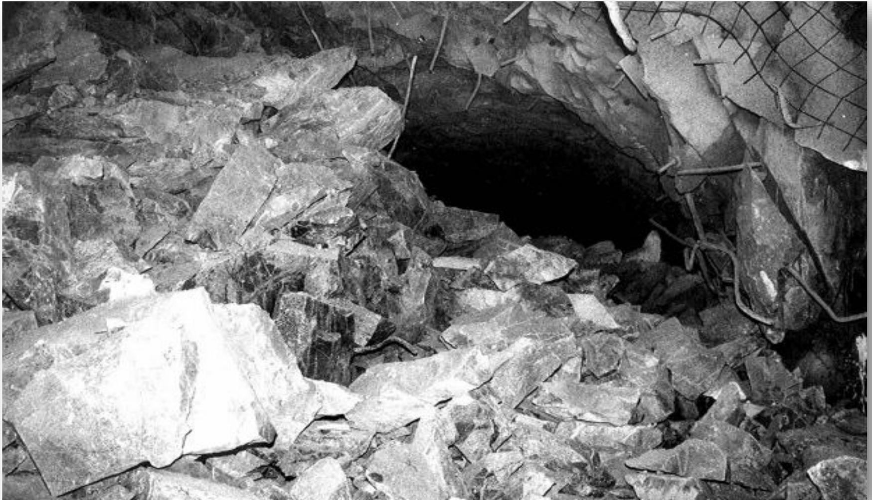
Typical rockburst damage, UCL drift, Ten sub 6 El Teniente (1991)
